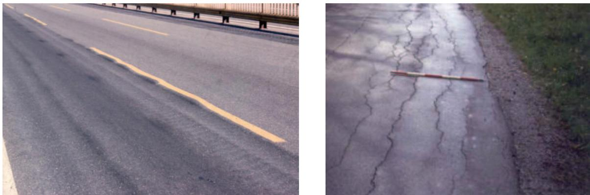
**Figure 1.** Damage of flexible pavements by rutting (left) and fatigue failure (right)
