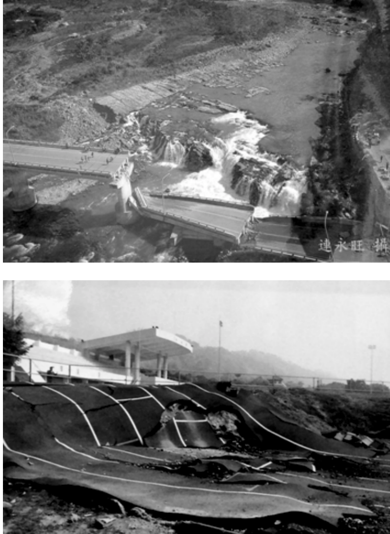
Fig. 1.4 Top panel: the bridge damage and scarp of 8 m height formed along the fault of the Chi-Chi earthquake on the river floor. Bottom panel: the fault scarp passing across the racetrack of one of the schools in Puli, Taiwan
