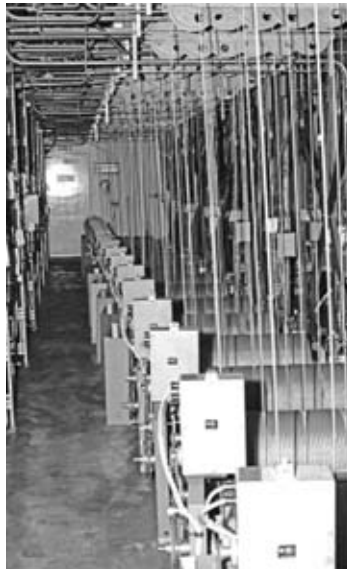
Figure 2.4 Winch floor showing the main winch drums and part of the pulley system
