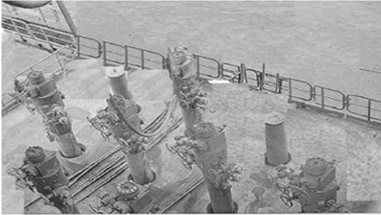
Figure 2.4. Production platform christmas tree and wellhead assembly
