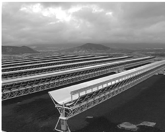
Fig. 1.11. The EUCLIDES demonstration power plant in Tenerife (1998) subsidized by the EU to industrialize the Madrid Prototype (1995). The mirrors were shaped aluminium plates covered with silvered acrylic film which cast 3.2\text{ W/cm}^2 on receivers including SATURN cells. The partners were ITER, BP Solar and UPM
