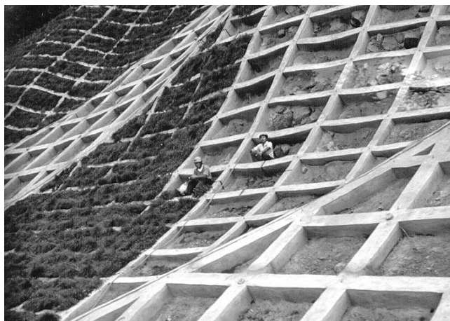
Figure A26 Road construction in Hokkaido, Japan. Much effort is made to stabilize the slopes, but landslides are common in Andosol areas.
