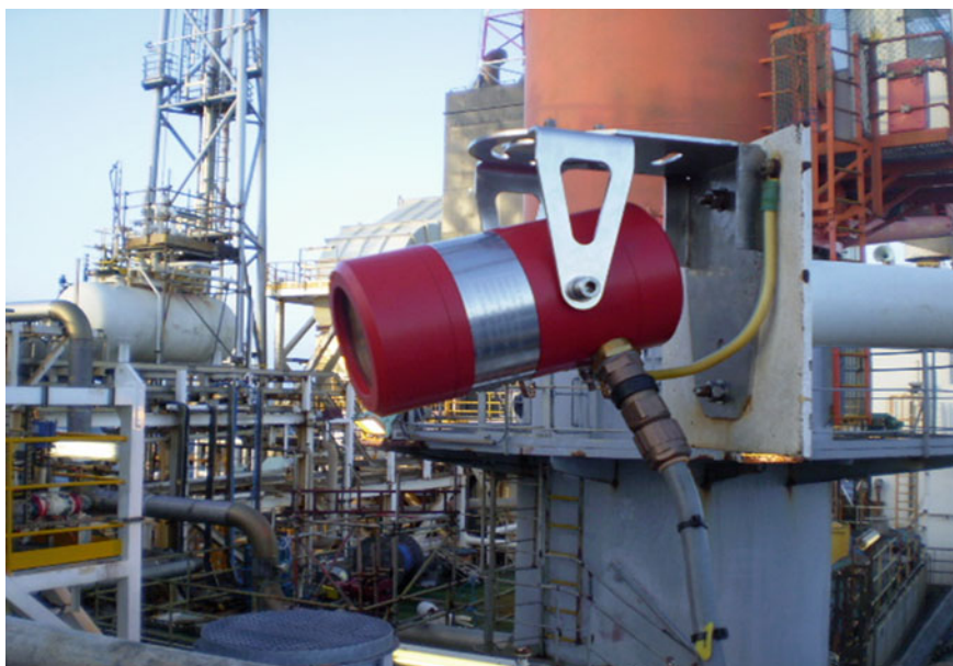
Fig. 2.2 Example of a spot-type flame VID device with camera and alarm processing in unit (courtesy of Micropack)
