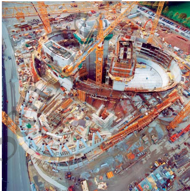
Fig. 11. Photo of the construction site. The trefoil principle is translated into concrete elements framing the horizontal floor plates
