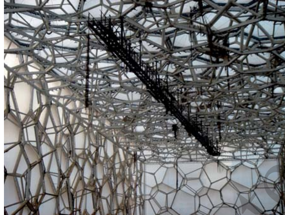
Fig. 2. The steel structure displays the 3-dimensional nature of the molecular structure of the Water Cube derived from foam bubbles
