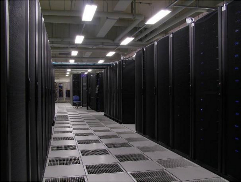
Fig. 1 Picture of the computer room. The blade servers and the RAID systems are mounted in the racks. A tape library system is placed at the far side.
