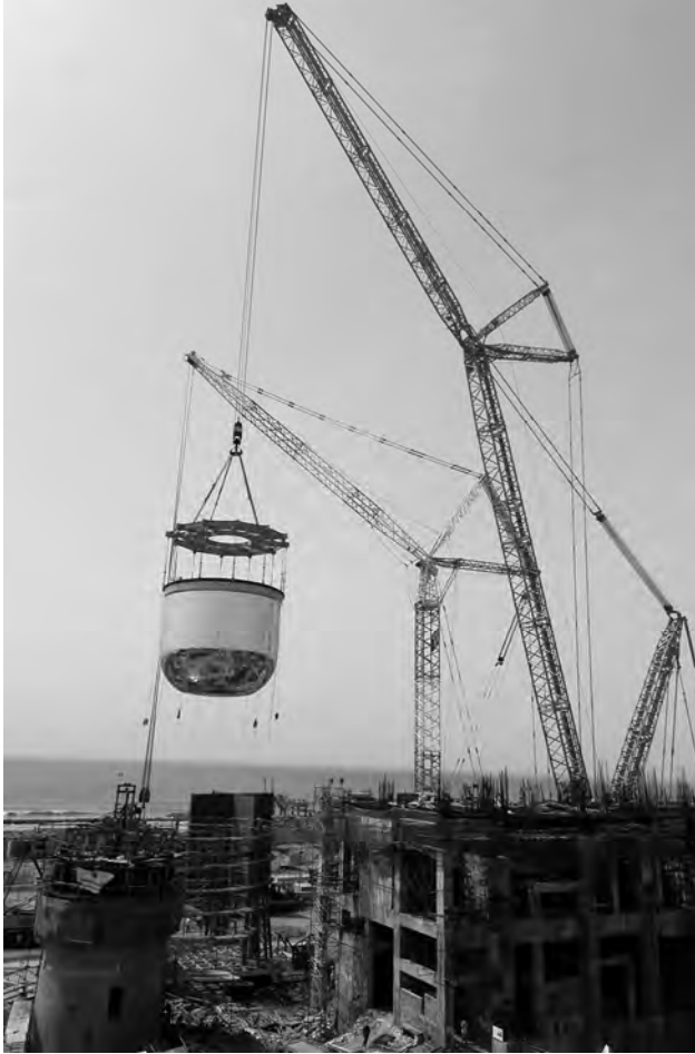
Figure 2.1. A crane lifts a nearly 200-ton nuclear reactor safety vessel at the Indira Gandhi Centre for Atomic Research at Kalpakkam, India, June 24, 2008. The reactor is a 500 MW prototype fast breeder and it is planned to begin commercial production by 2011. (Photo: Babu/Reuters/Scanpix)
