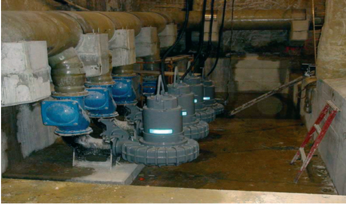
Figure 2.6 Typical pumping station for a reservoir. Taken from CLABSA (2007)
