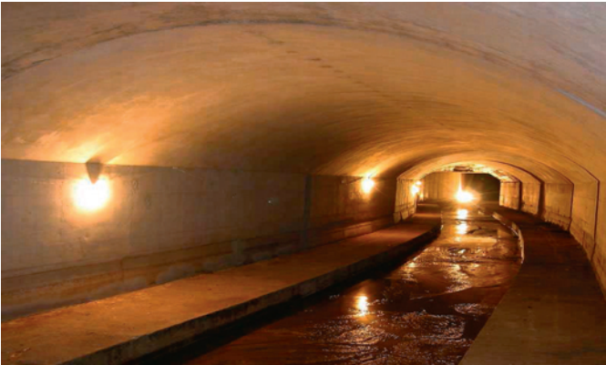
Figure 2.2 Large-diameter sewer. Taken from CLABSA (2007)
