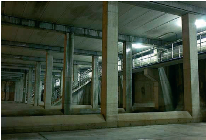
Figure 2.3 Inside a retention tank. Taken from CLABSA (2007)
