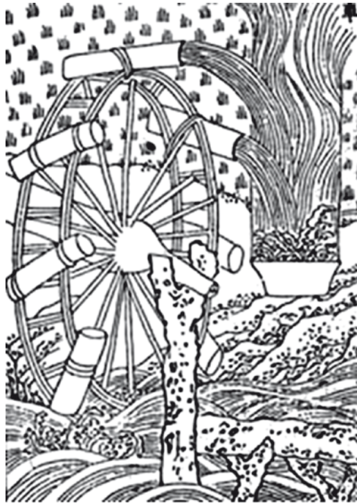
Fig. 2.8 Bamboo water wheel (From the Nong Shu [86,141])
