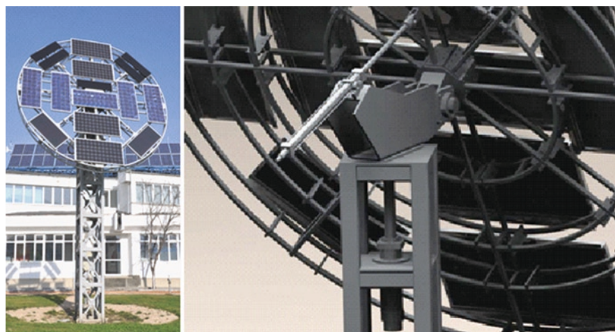
Fig. 2 PV tracked platform installed in the Transilvania University of Brasov
