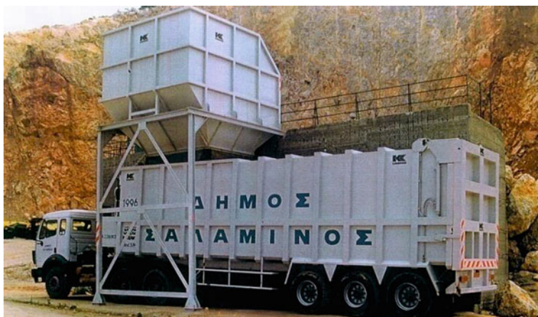
Fig. 2 Transfer station with a ramp, a hopper and a semitrailer under the hopper in loading position
