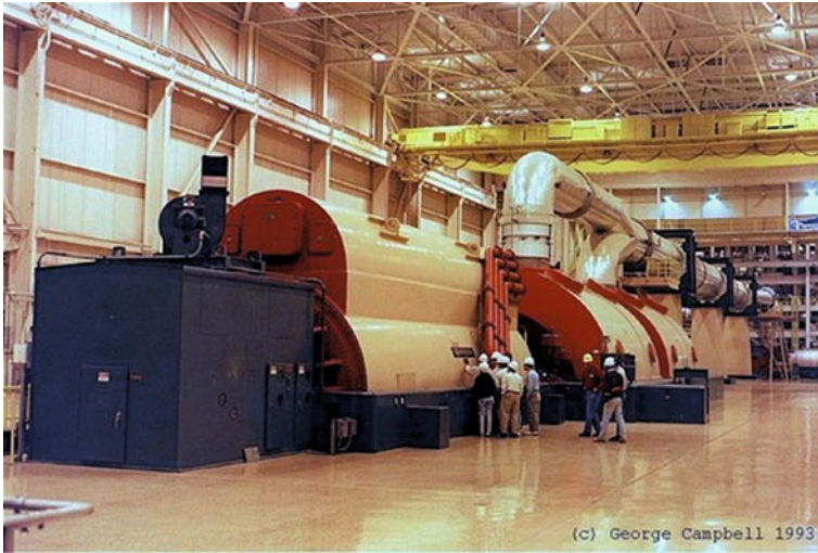
Fig. 2.1 750 MW generator with 2 steam turbines. From Campbell G (1993)
