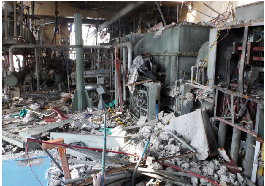
Fig. 2.11 Some of the nuclear plants at the coastline were hit, and the reserve system for cooling in case of an incident was destroyed, leading to overheating of the plant and leakage of radioactive material. Picture from Fukushima nuclear plant (Photo Scanpix, with permission)
