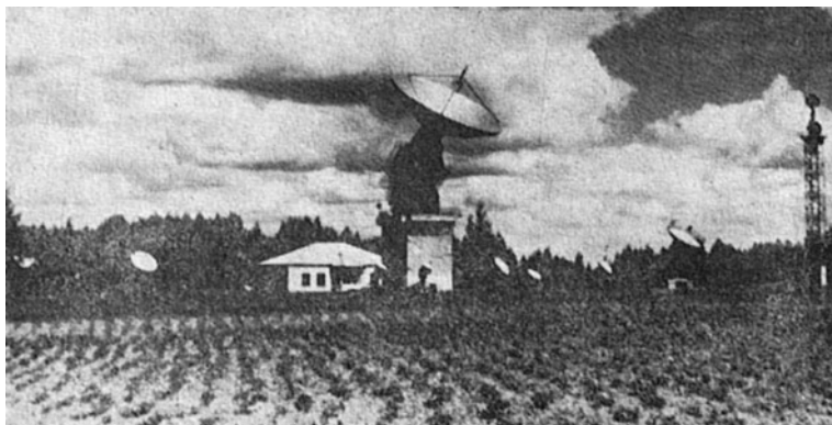
Fig. 2.4 15-m radio telescope, the system of smaller radio telescopes, and the black disk for the solar service at Zimenki
