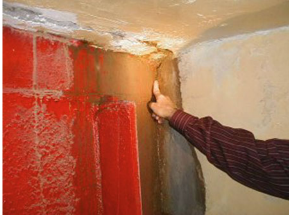
Fig. 2.11 Crack in concrete at draft tube door
