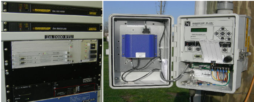
Fig. 2.19 Example station and feeder voltage/VAR control devices
