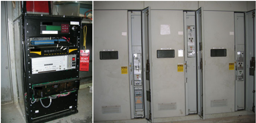
Fig. 2.8 Typical substation controller and vault switch
