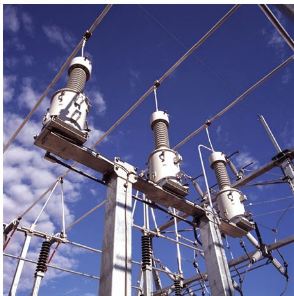
Fig. 2.27 Outdoor switchgear busbar (upper conductors) with voltage transformers (Courtesy of General Electric)
