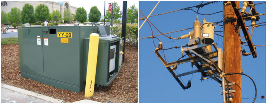
Fig. 2.7 Typical pad-mount and pole-mount switches
