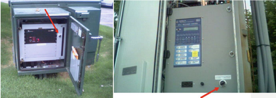
Fig. 2.6 Pad-mount controller and pole-mount reclosing relay with enable/disable switches
