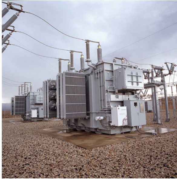
Fig. 2.26 Voltage transformers (Courtesy of General Electric)
