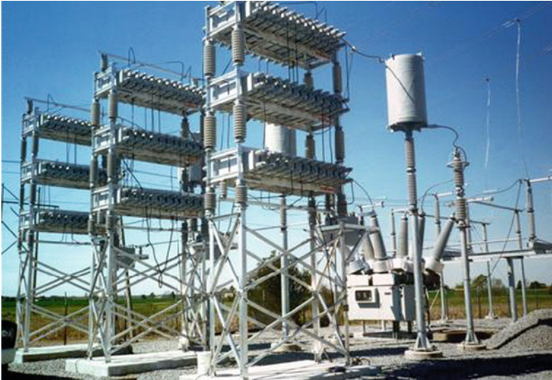
Fig. 2.31 Capacitor Bank (Courtesy of General Electric)
