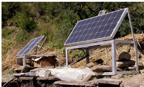
Fig. 2.18 A solar PV cluster system for up to 12 homes. One 75 W p PV module ( right side ) generates power which is stored in the battery-bank installed inside the home. All other cluster homes are connected through underground cables to the battery-bank, which provides up to 3 days of power without sunshine
