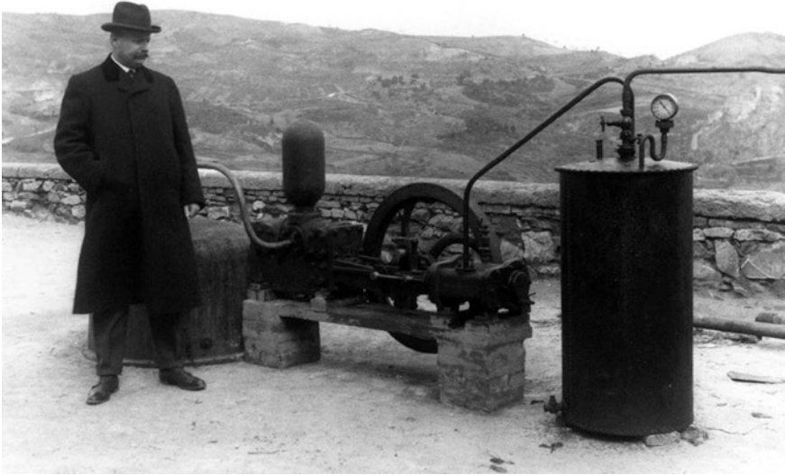
Fig. 2.4 Lardarello 1904: The picture shows Principe Piero Ginori-Conti with his apparatus that converted geothermal to electrical energy for the first time in history. The installation had the power to light five light bulbs (Photograph: Unione Geotermica Italiana 2010)
