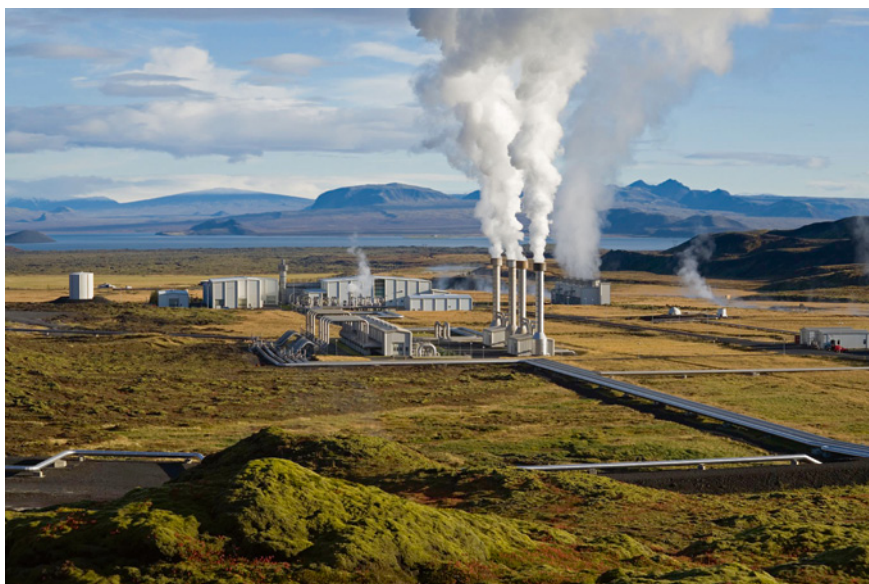
Fig. 2.5 Nesjavellir Power Plant on Iceland; 120 MW electrical power plus 380 MW thermal power from 83 °C water in 2010, reservoir temperatures up to 380 °C (sources http://de.academice.ru/dic.nsf/dewiki/1010201 and http://www.or.is/media/PDF/Nesjavellir%20ENS%2007.pdf )
