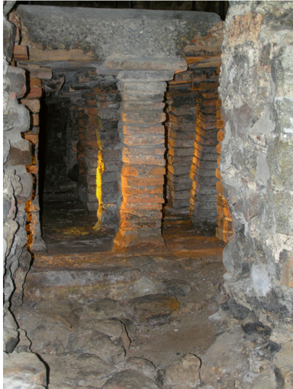
Fig. 2.3 Thermal spa Baden–Baden, Roman soldier spa, underfloor heating system, first geothermal heating system
