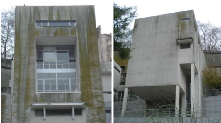
Fig. 1 ETICS defacement due to biological growth (bulking located in porto - Portugal)
