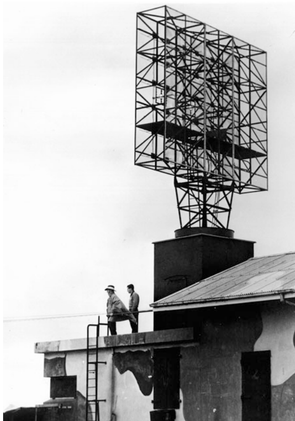
Fig. 2.15 The 200 MHz shore defence radar at Dover Heights in Sydney during World War II. In the post-war era the antenna was converted to a radio telescope with no transmitter. In early 1946 this antenna was used for groundbreaking solar radio observations by Payne-Scott, Pawsey and McCready (Chap. 7). Payne-Scott carried out the first radio astronomical interferometry with this antenna on 26 January 1946 (Australia Day) at sunrise. See Fig. 7.2 (Copy obtained from the collection of W.T. Sullivan. Original from CSIRO Radio Astronomy Image Archive)
