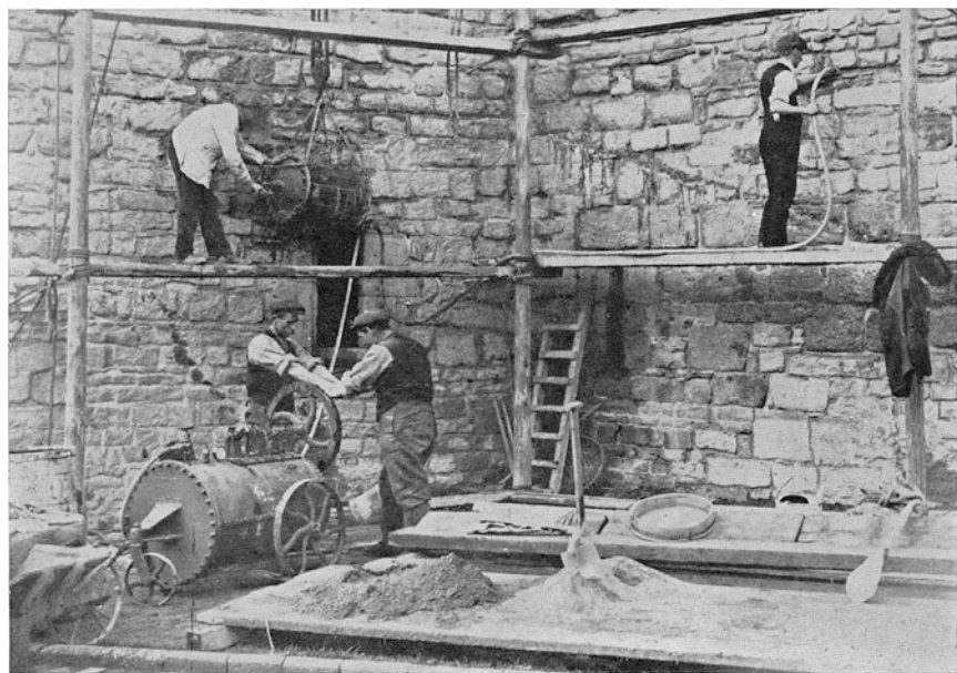
GROUTING MACHINE AT WORK (SEE PARA. 147).
