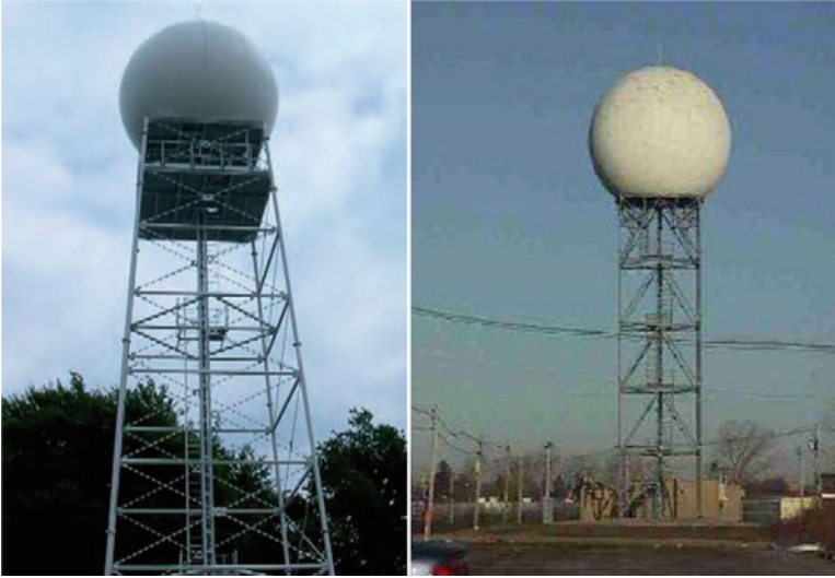
Fig. 2.4 Example of a Met Office C-band weather radar in the UK ( left ) and a NOAA/National Weather Service S-band (NEXRAD) radar in the USA ( right ) (Met Office 2009: Contains public sector information licensed under the Open Government Licence v1.0, and courtesy: National Oceanic and Atmospheric Administration http://www.erh.noaa.gov/ )
