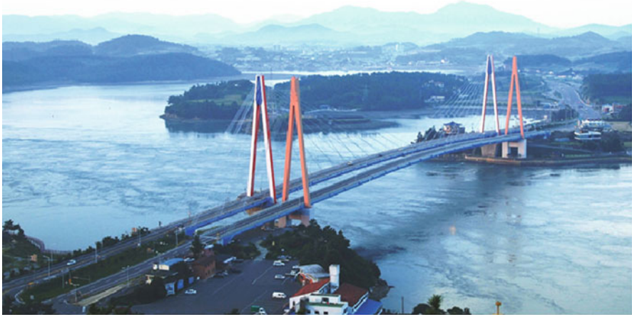
Fig. 2.38 Densely instrumented cable-stayed 2nd Jindo Bridge in South Korea uses wireless sensors (Photo courtesy of B. Spence, 2011)
