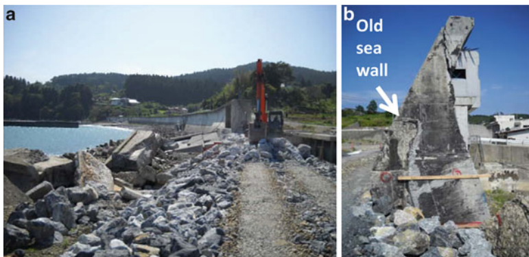
Fig. 2.11 Photos of seawalls with improvements prior to the tsunami. (a) Damaged sea walls in Ofunato City. (b) Evidence of improvements
