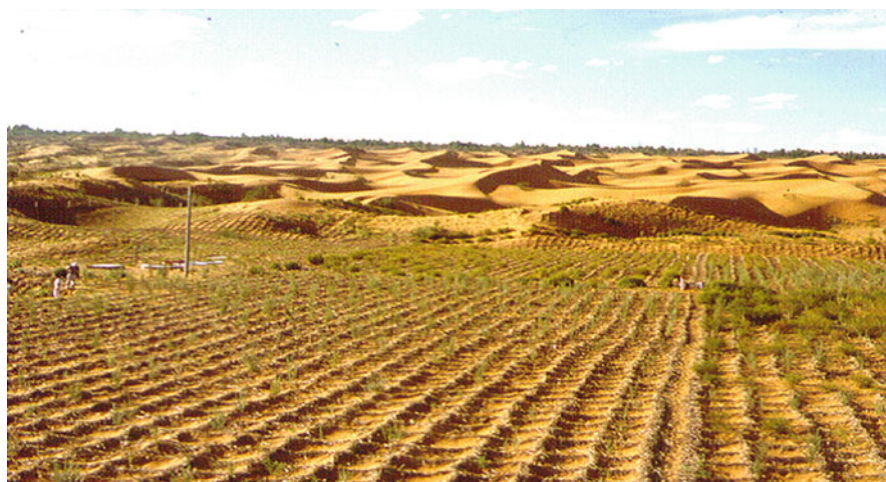
Fig. 2.22 A view of part of the Shapotou Desert Research Station showing the system of checkerboards made with straw to increase surface roughness and reduce sand movement
