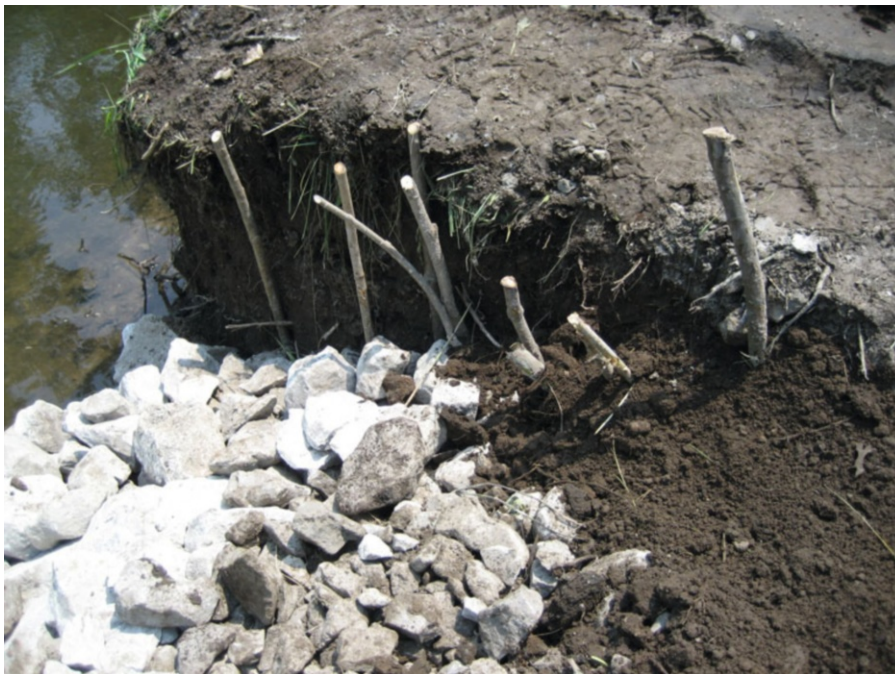
Fig. 4 Placement of willow poles in keyway
