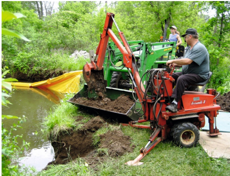
Fig. 3 Construction of keyway for a rock vane
