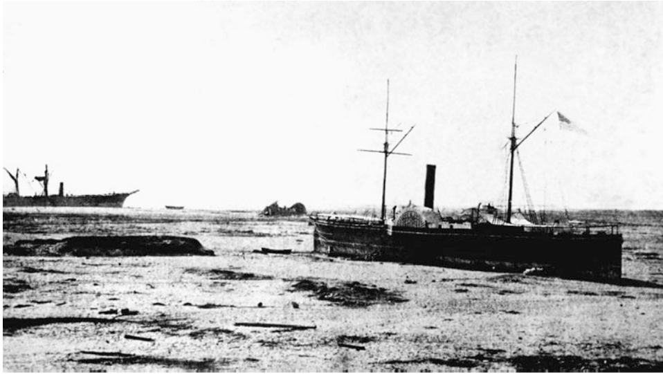
Fig. 2.11 The American warship Wateree in the foreground and the Peruvian warship America in the background. Both ships were carried inland 3 km by a 21 m high tsunami wave during the Arica, South American event of August 13, 1868. Retreat of the sea from the coast preceded the wave, bottoming both boats. The Wateree, being flat
