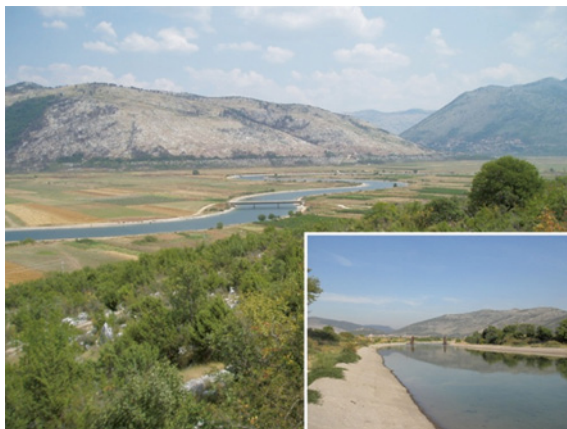
Fig. 18 River Trebišnjica, BiH. River bed covered by shotcrete
