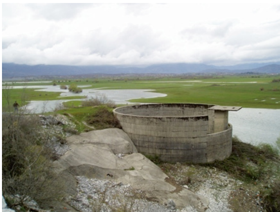
Fig. 21 Nikšić Polje, Montenegro. Cylindrical dam around a large estavelle at the reservoir bank
