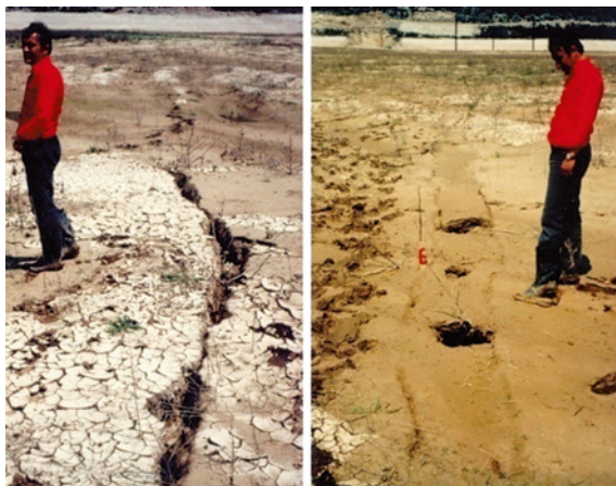
Fig. 11 Hutovo Reservoir, BiH. Ponors and large cracks created during the first reservoir filling
