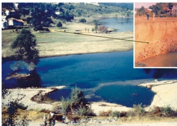
Fig. 12 Mavrovo Reservoir (FYUR Macedonia). Collapses as a consequence of reservoir operation
