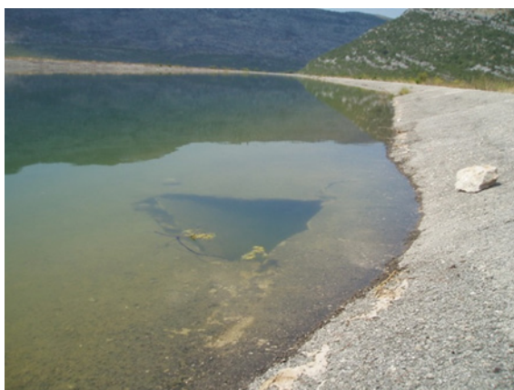
Fig. 13 Demolished shotcrete at the reservoir bank
