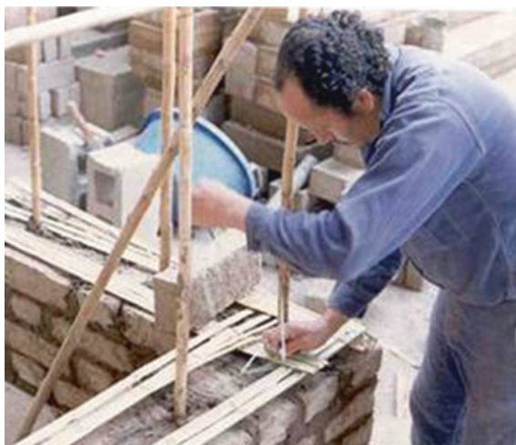
Fig. 27 Internal cane mesh reinforcement [77]
