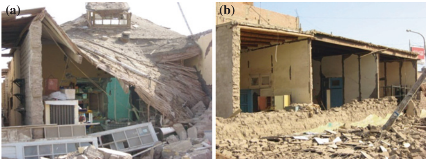
Fig. 8 Collapse of adobe houses during the Pisco earthquake in 2007, Peru. a Roof supported on the façade walls. b Roof supported by transversal walls
