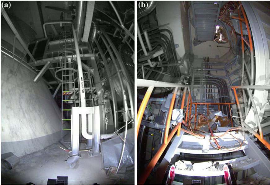
Fig. 1 High-resolution photos captured in the reactor building of unit 3. The left shows the piping of the core spray system and the right shows the rubble blocking the staircase to the third floor
