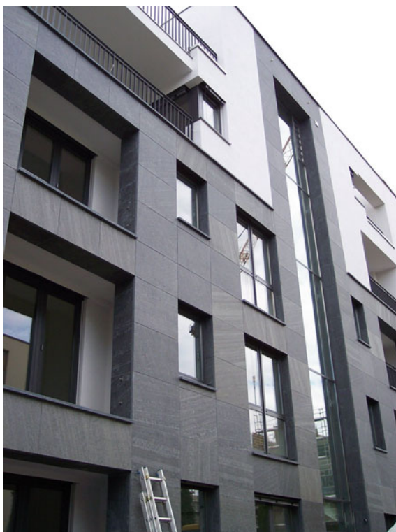
Fig. 2.48 Building cladded with the Knotenschiefer (knotted slate) of Theuma. The very specific decor is due to the contact metamorphic overprint, which had produced the mineral growth (Natursteinwerk Theuma AG, Theuma in Germany)
