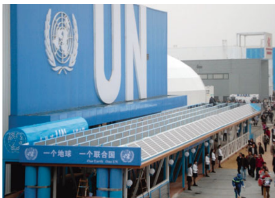
Fig. 2.10 Integrated solar thermoelectric system on the top of the waiting area of the UN Pavilion
