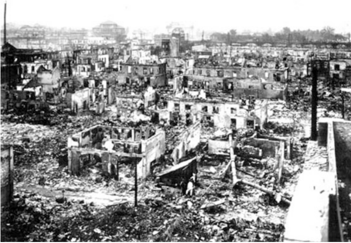
Fig. 2.2 Damage to modernistic buildings by 1923 Kanto earthquake (home page of the National Science Museum)
