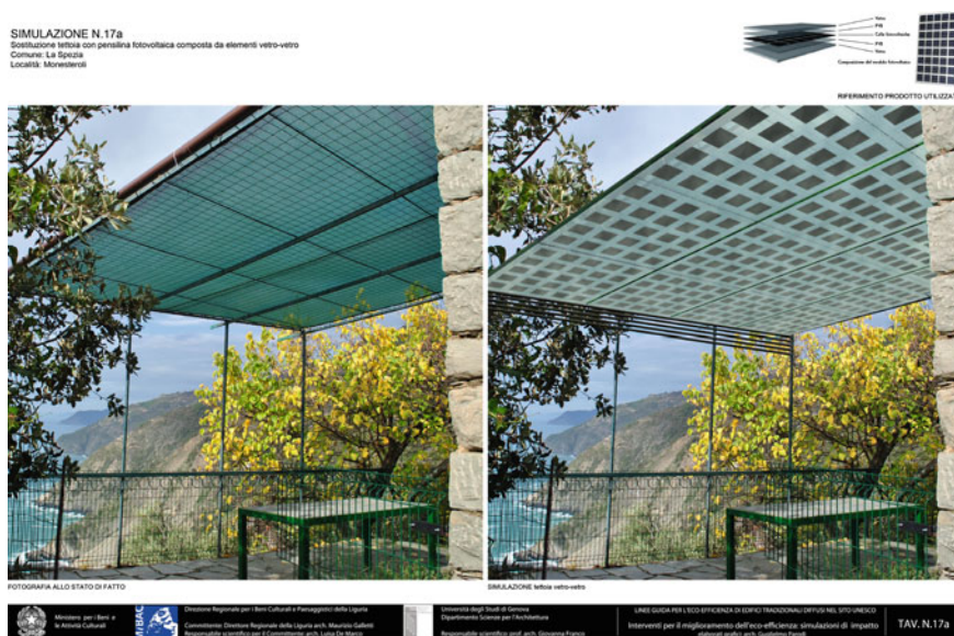
Fig. 8 Photo simulation of the substitution of a plastic shelter with PV glass cells
