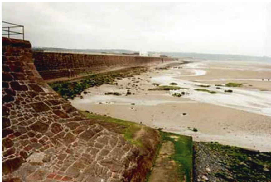
Fig. 2.18 The sea wall at St Ouen's Bay, Jersey, with the beach lowered by reflection scour. © Geostudies
