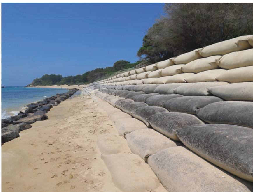
Fig. 2.11 A sandbag rampart marks the site of beach erosion at Portsea, Port Phillip Bay, Australia, in 2013. © Geostudies
