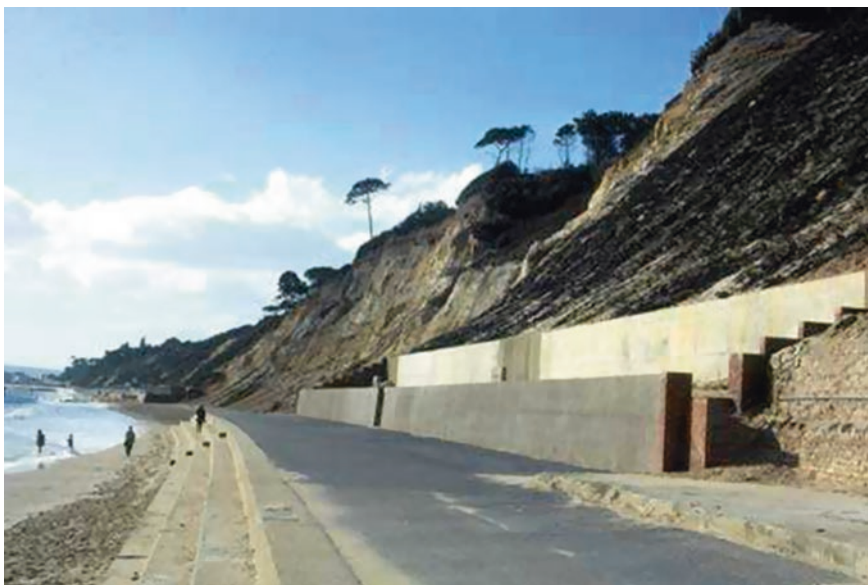
Fig. 2.4 Canford Cliff after the construction of a concrete esplanade along the base of the cliff. This halted marine erosion, but also reduced the supply of sand and gravel to adjacent beaches, which became depleted by marine erosion. © Geostudies
