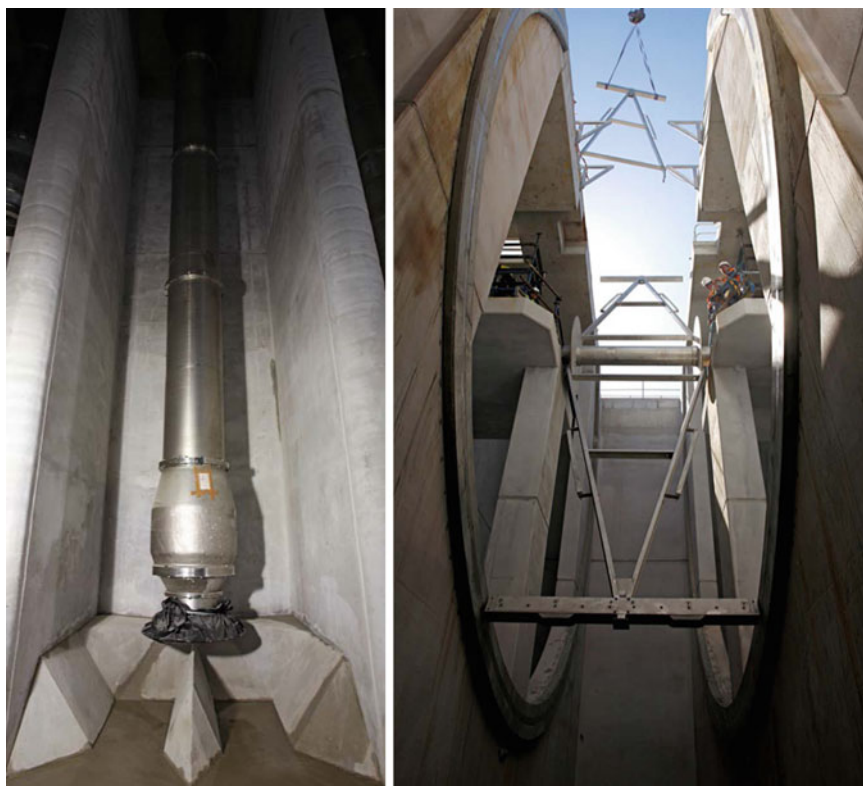
Fig. 2.13 SDP intake pump/fine screen during installation
