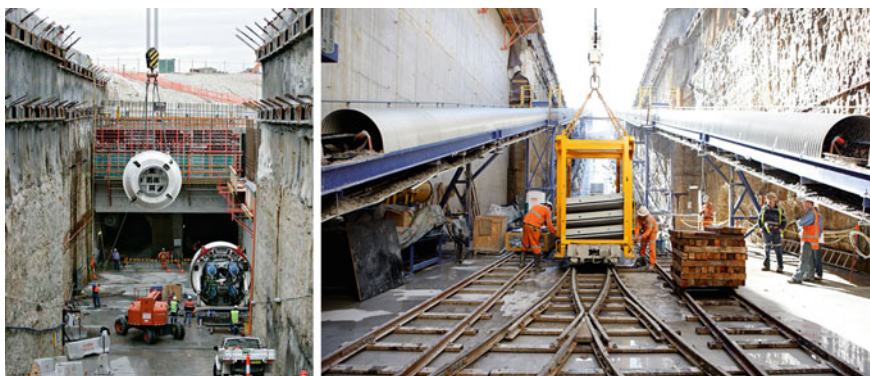
Fig. 2.11 TBM assembly within the “box-cut” leading to the tunnel portals/haulage railway and spoil conveyors leading out of the “box-cut”
