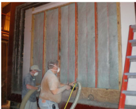
Fig. 2.5 PCM-enhanced materials used as an integral part of the building thermal envelope. Right picture shows construction of an experimental double wall with exterior layer of cavities containing PCM-cellulose insulation
