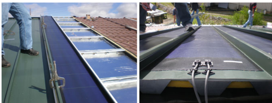
Fig. 2.16 Construction of the experimental PCM-PV roof—Oak Ridge, TN, USA
