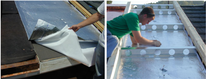
Fig. 2.14 Construction details of a roof assembly containing, reflective insulation, and subventing air channels, followed with two PCM insulation systems produced by Outlast, USA (PCM-enhanced foam and PCM-impregnated fabric, see left photograph )
