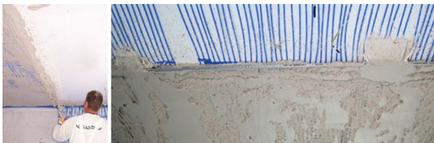
Fig. 2.13 Installation of the active-chilled ceiling system containing PCM-enhanced plaster and plastic micro-tubing. Fraunhofer ISE, Germany ( http://www.ise.fraunhofer.de/en/areas-of-business-and-market-areas/energy-efficient-buildings/hot-and-cold-storage )
