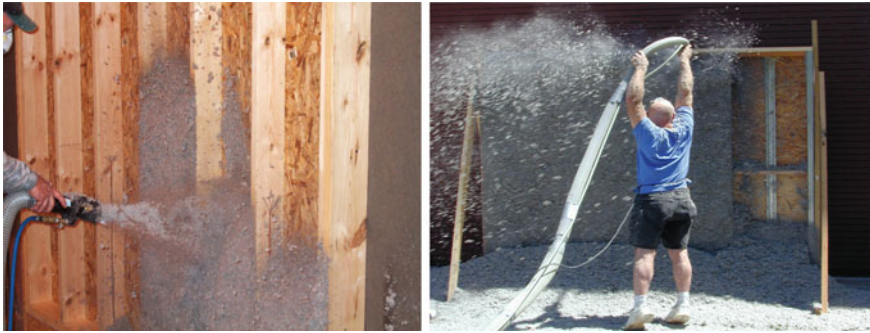
Fig. 2.7 Installation of PCM-enhanced cellulose in the test walls
