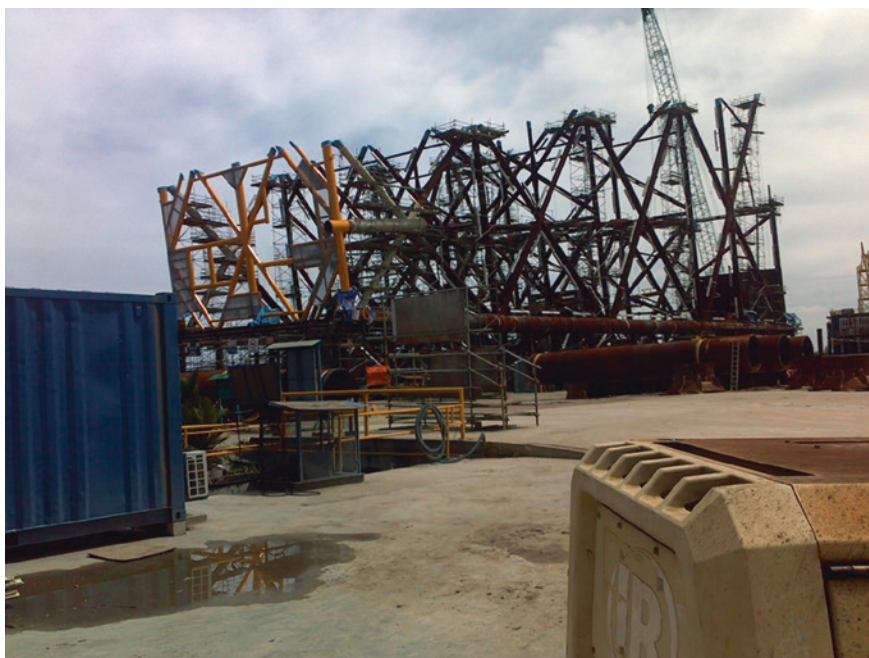
Fig. 2.1 Jacket platform under fabrication at a yard
