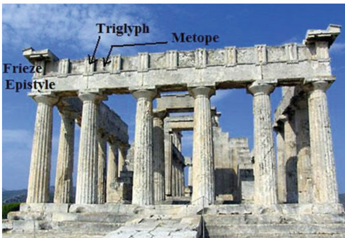
Fig. 2 View of the Temple of Aphaia, in Aegina, Greece. Its monolithic, free-standing columns support massive epistyles and the frieze atop and the entire rocking frame remains standing for more than 2500 years in a region with high seismicity
