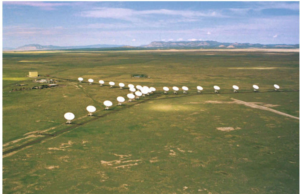
Fig. 1.26 The Very Large Array (VLA) in New Mexico consists of 27 antennas with a diameter of 25 m each that can be moved on rails. It is used in four different configurations that vary in the separation of the telescopes; switching configurations takes about 2 weeks. Credit: NRAO/AUI
