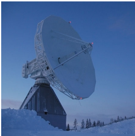
Fig. 2.6 TTCF S-band 11 m dish antenna (courtesy of ESA)
