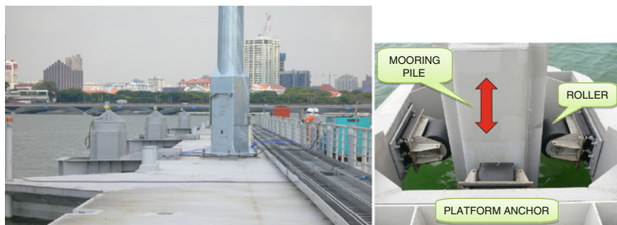
Fig. 8 Detachable mooring system
