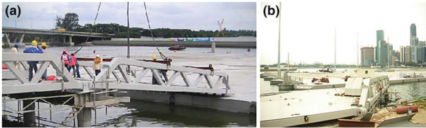
Fig. 22 a Erecting the truss girders and b installing the deck panels
