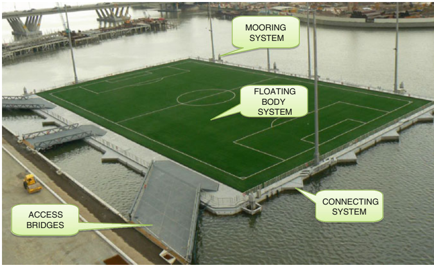
Fig. 4 System description of floating performance stage at Marina Bay
