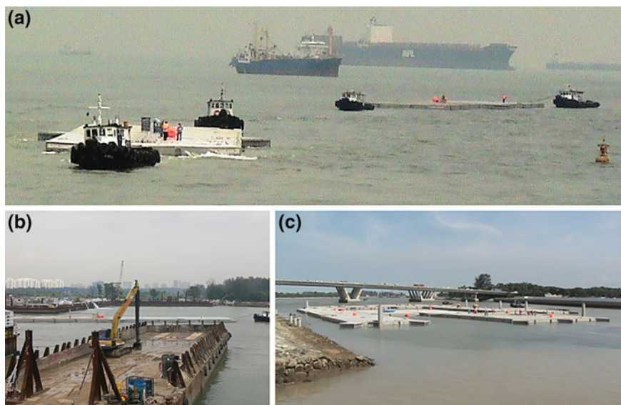
Fig. 21 a Pontoons being towed by tug boats. b Passing through the Marina Barrage. c Arriving and assembly of floating pontoons on-site
