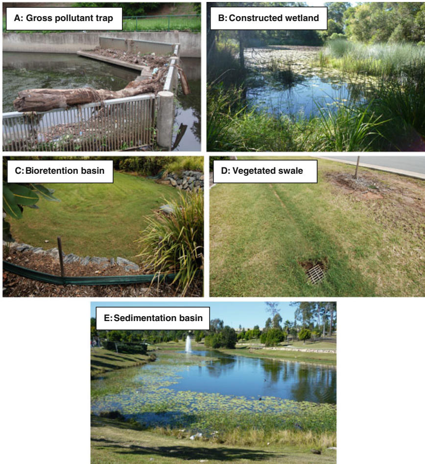
Fig. 2.1 Typical structural stormwater treatment systems a gross pollutant trap b constructed wetland c bioretention basin d vegetated swale e sedimentation basin
