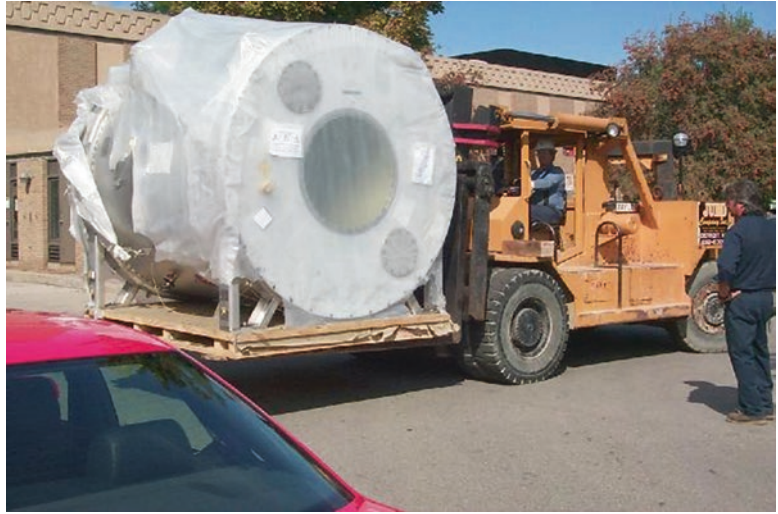
Fig. 9 A 3T magnet during installation at the University of Michigan's FMRI Laboratory
