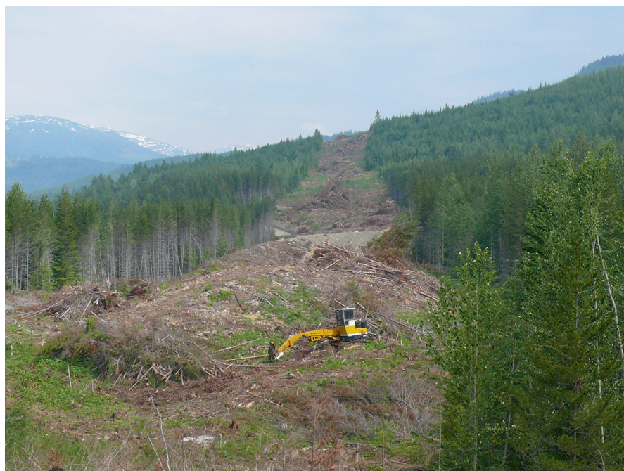
Fig. 2.2 The 287 kV Northwest Transmission Line, under construction in this image, will stretch 344 km across an undeveloped but mineral-rich region of northwestern BC (Photo by C. Johnson). The transmission line will provide electricity to planned and future mines as well as an interconnection point for run-of-river hydroelectric development. The right-of-way and associated infrastructure (effects) will have direct impacts on biodiversity and other values. More complex, however, are the indirect economic growth-inducing effects resulting from the provision of inexpensive electricity to large industrial projects. The positive and negative impacts of future resource development will greatly exceed the impacts of the transmission line; however, those impacts are difficult to predict and consider during project assessment and approval
