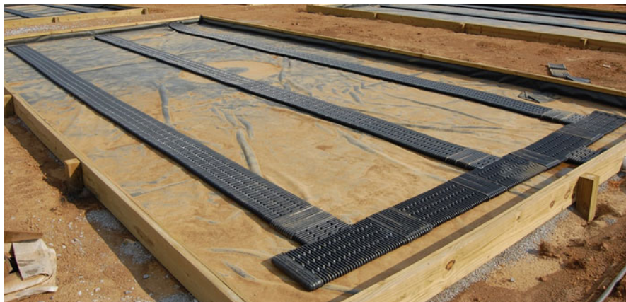
Fig. 2.31 Flat panel tile being used instead of the traditional round perforated tile. Flat panel tile is laid on the subgrade and not imbedded into it saving trenching and spoil disposal costs
