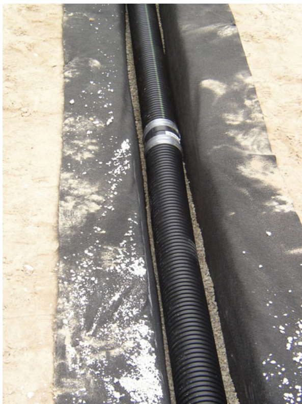
Fig. 2.15 Four inch in perforated tile placed into the subgrade and back-filled with gravel to help facilitate subsurface drainage
