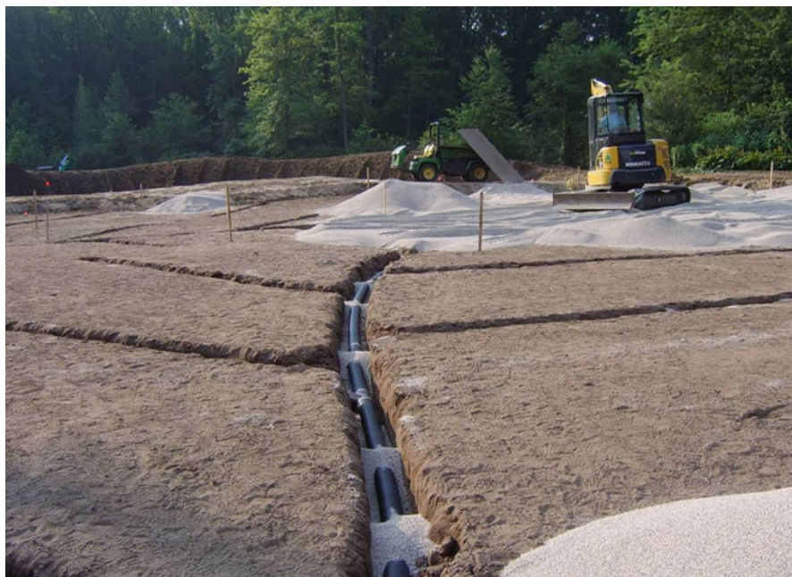
Fig. 2.26 Trenches in golf green subsoil with drainage tile and being backfilled with gravel
