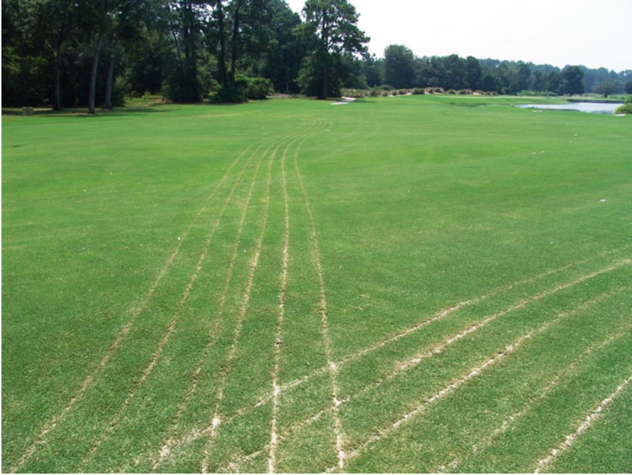
Fig. 2.24 Narrow slit drains backfilled with sand to reduce surface moisture. This helps lower the water table until the slits fill with water
