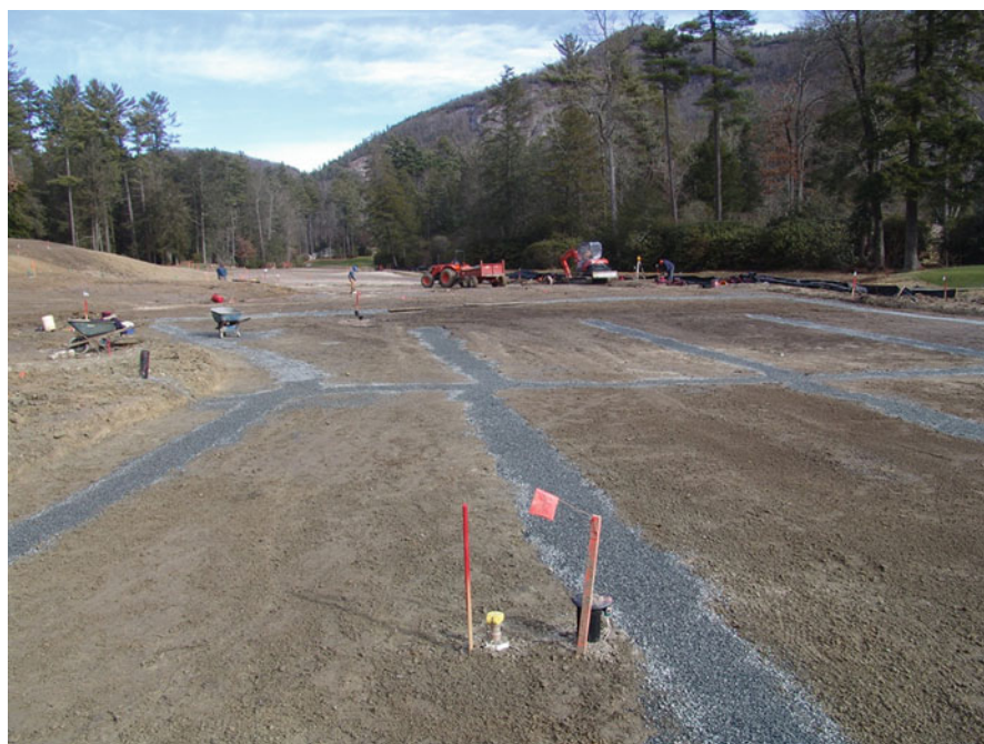
Fig. 2.34 Subsurface drainage being installed on a golf course fairway. Drainage ditches are back-filled with gravel prior to soil placement
