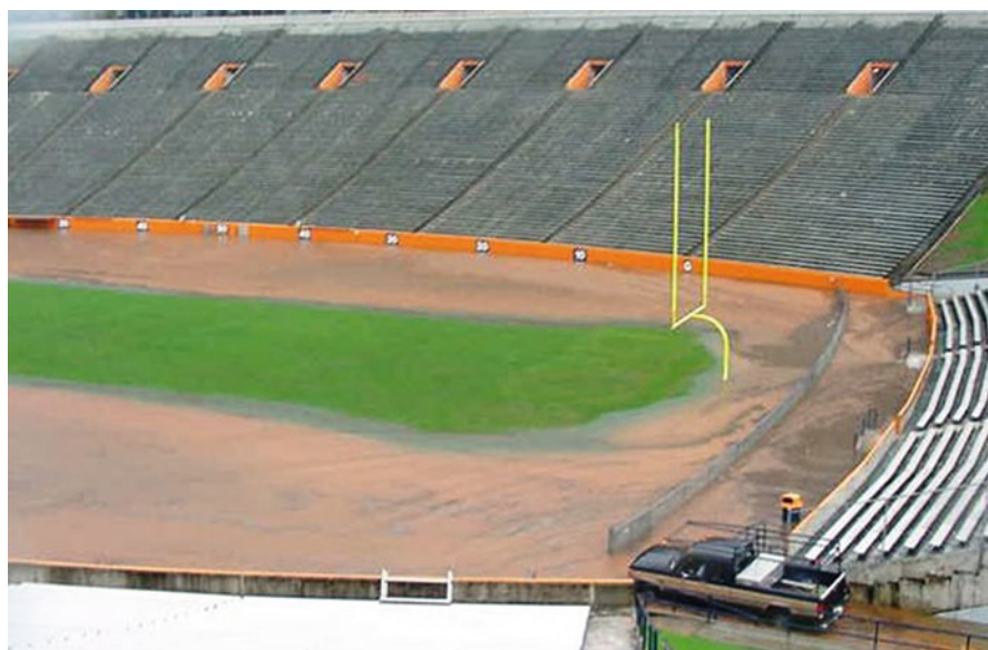
Fig. 2.11 “Bathtub” effect of inadequate surface and subsurface drainage due to underlying clayey soils without sufficient drainage and outlets for the amount of rainfall received
