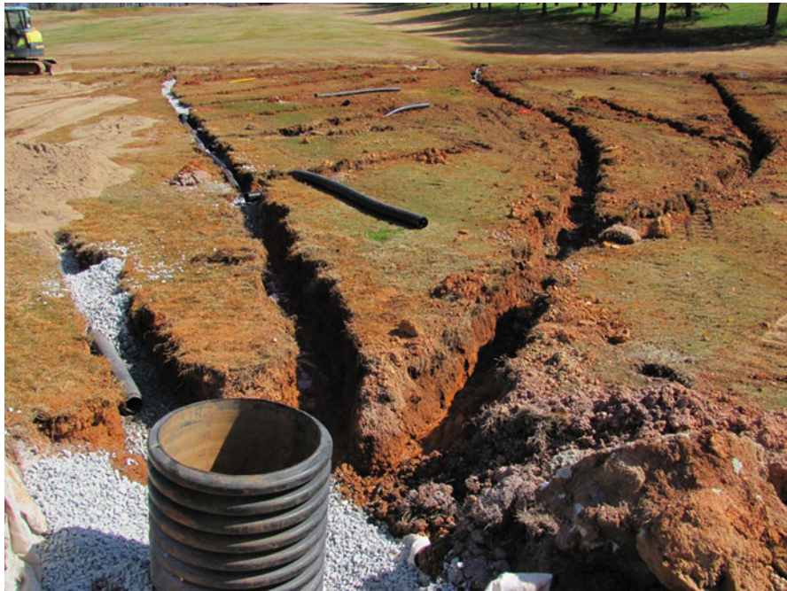
Fig. 2.38 Collection point for several main lateral drainage lines. The collected water is then removed or redistributed away from the property
