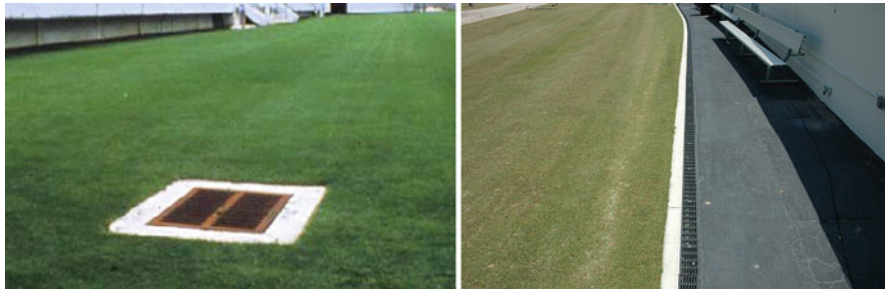
Fig. 2.45 Traditionally used surface catch basis to capture excessive surface water ( left ); strip surface drains to capture excessive surface water ( right )
