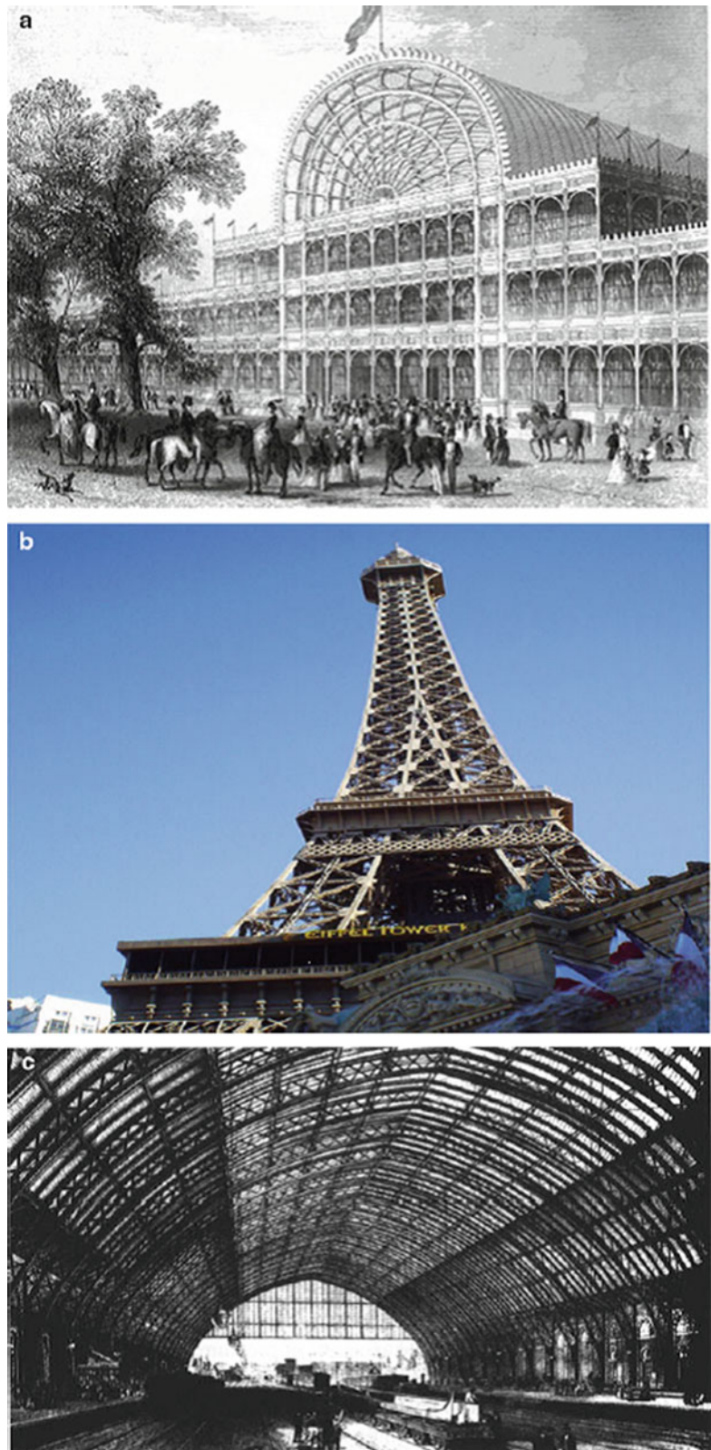
Fig. 2.10 Examples of structures made of iron trusses. (a) Crystal Palace. (b) Eiffel Tower. (c) Saint Pancras station
