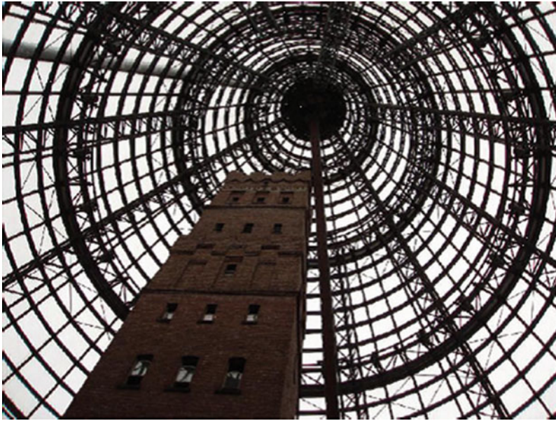
Fig. 2.13 Three-dimensional truss roof system
